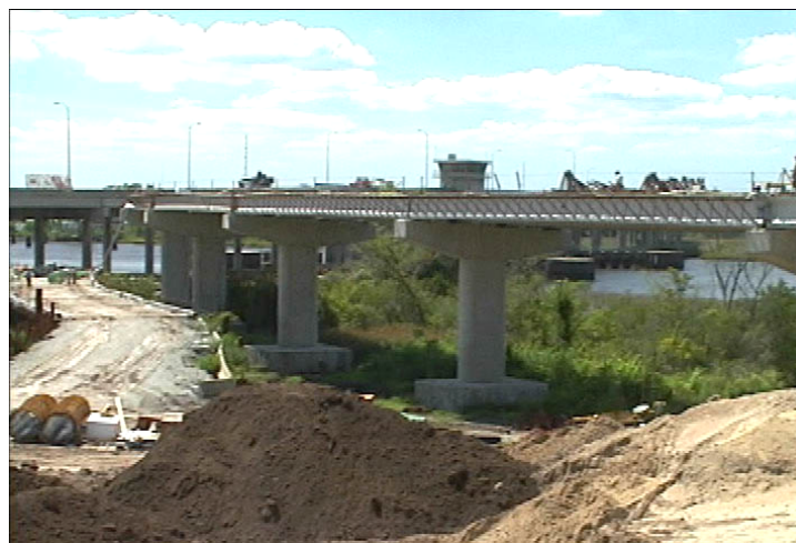
Martin Luther King, Jr. Parkway Construction 2003
