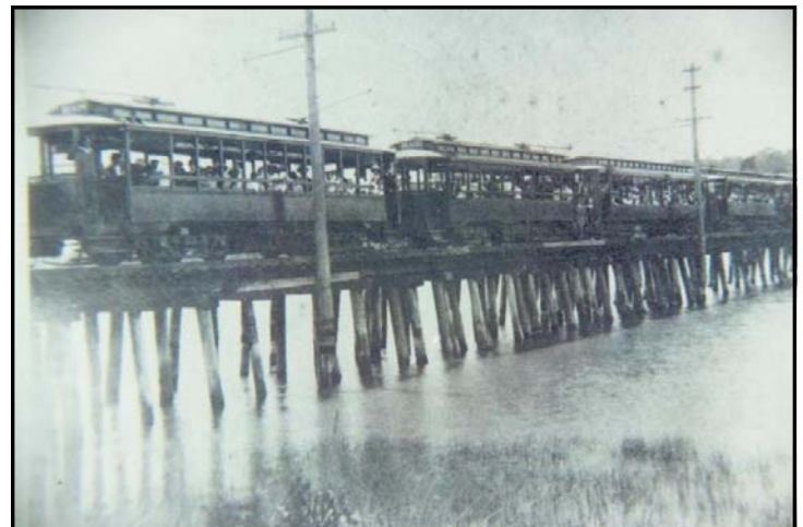
Train cars on the Bradley Creek trestle circa 1915
