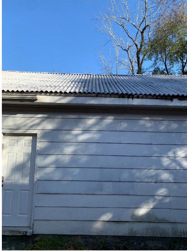
106 North 6 th Street | Looking north at garage siding and metal roof | 2/2022 (staff)
