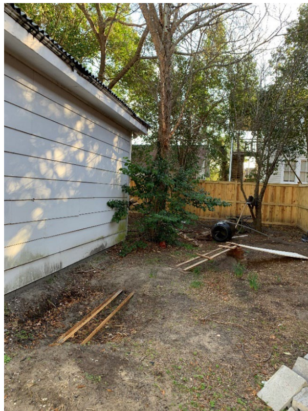
106 North 6 th Street | Looking east at garage siding and back yard | 2/2022 (staff)
