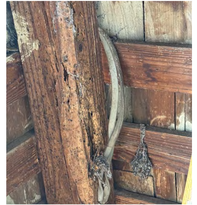
Termite damage to interior Structure
