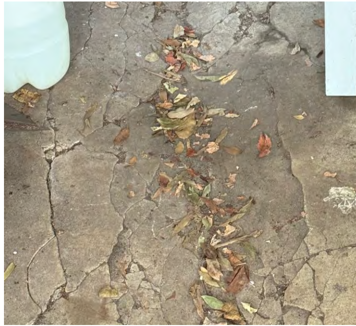
Broken Slab/garage Floor
