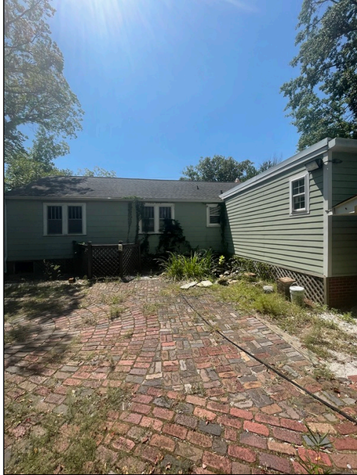
9 - View of the non-ACM fiber cement straight lap siding on the back addition.
