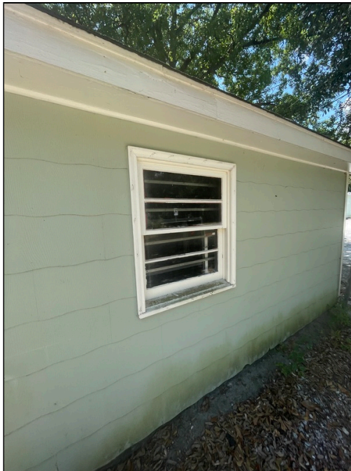
8 - View of the asbestos -containing wavy fiber cement siding on the shed.
