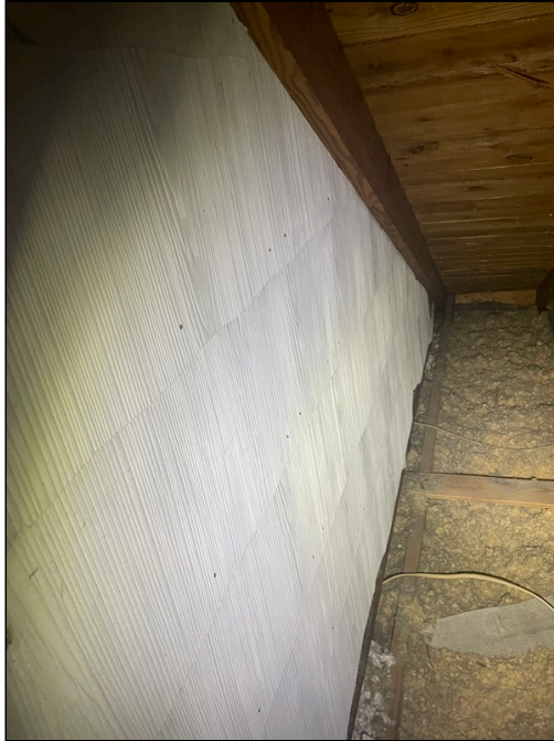
7 - View of asbestos-containing cement siding in the attic.
