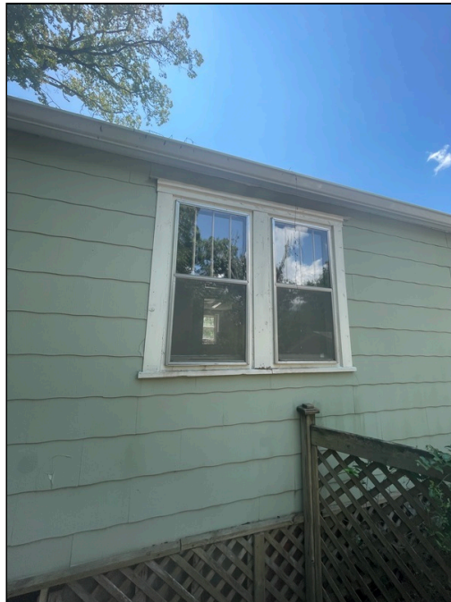
6 - View of the asbestos-containing wavy fiber cement siding on the house.
