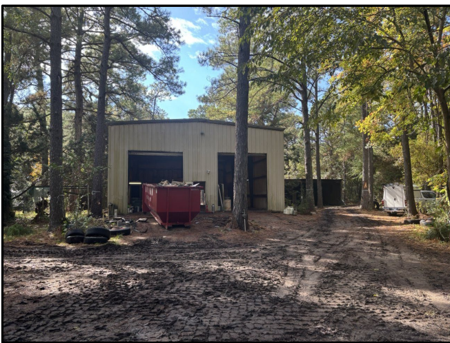
Photo of two of the storage structures
