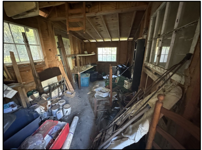
Interior of the shed abutting the residential structure on Tract 3.
