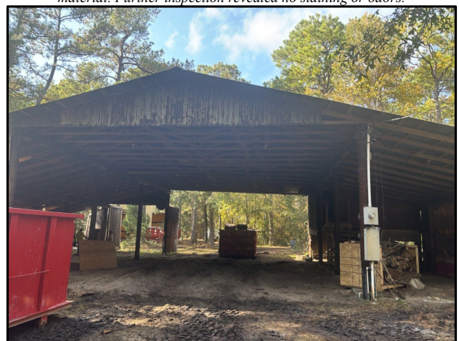
General photo of the interior of one of the storage structures
