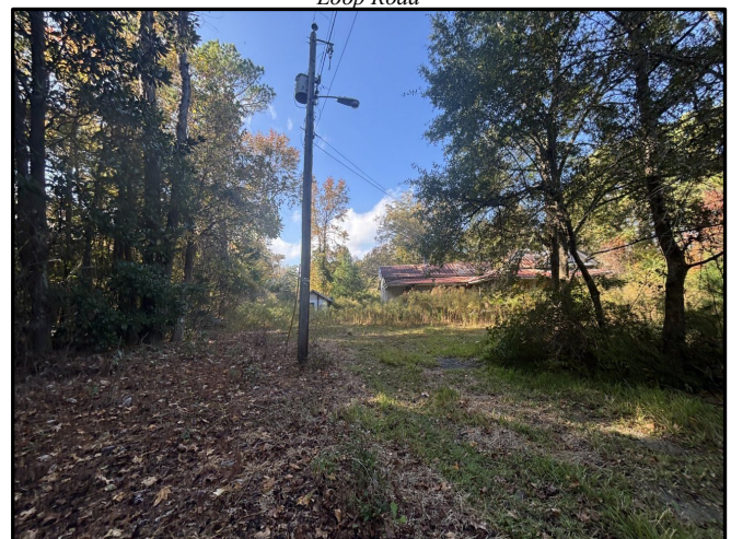
Standing at the entrance to Tract 3, facing the single-family residential structure; picturing the overhead electric line and transformer
