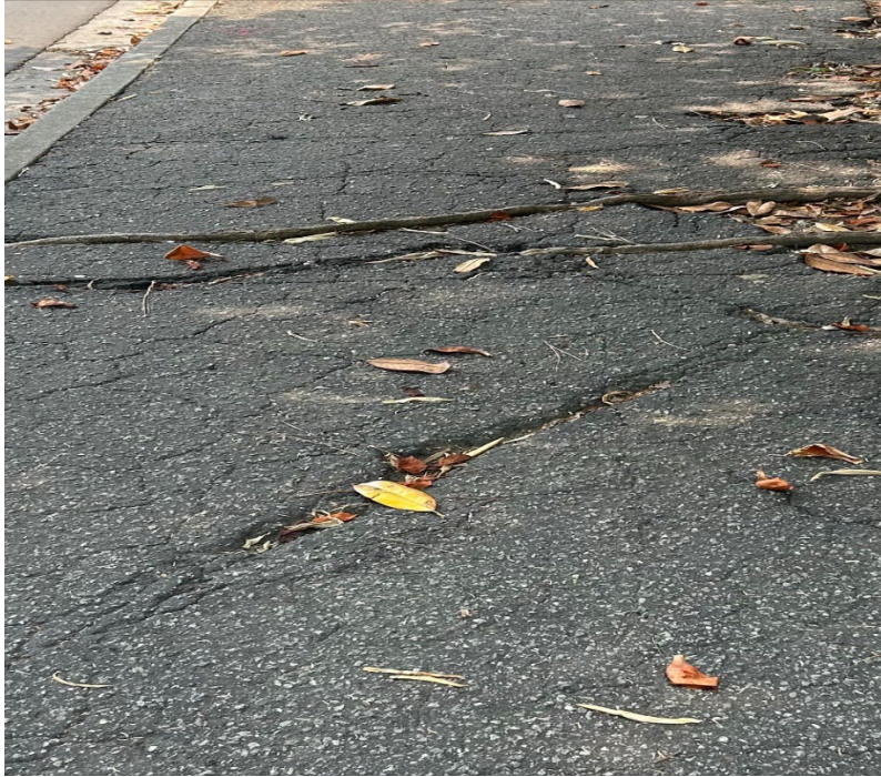
Image 2: Typical section condition
