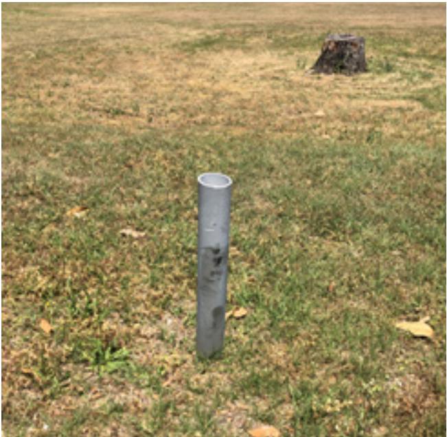
⚡ PVC stub in open field at Archie Blue should be removed to prevent safety concerns
