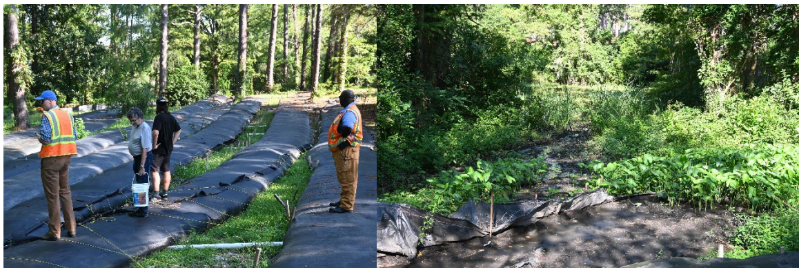
Plate 1a. (left) Array of Geotubes holding dredged sediment on shore near Squash Branch, August 2024, Plate 1b (right) Severe drainage from Geotubes passing through sediment fencing toward the lake, caused by heavy rains.
