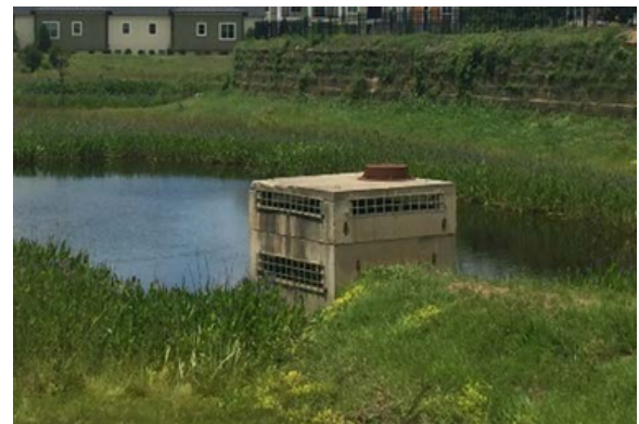
All stormwater wetlands should have an outlet though the design may differ (Photo Credit: Hunter Freeman)
