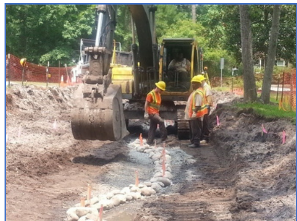
Channels may require added river rock or other soil modifications (Photo Credit: City of Wilmington)
