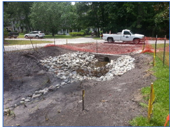
Example of an inlet during construction (Photo Credit: City of Wilmington)
