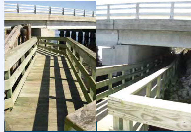
Pedestrian walkway under Corbett Ave (NC 24) in Swansboro, NC
