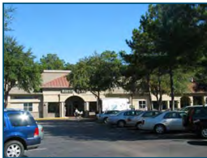
Interest-added architectural design and mature interior lot landscaping
