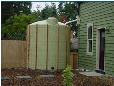
Cistern to collect rainwater for future use
