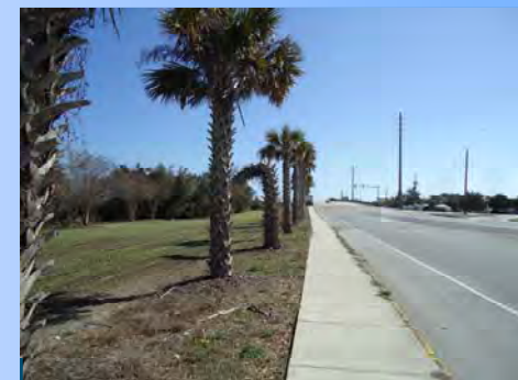
Wrightsville Avenue looking east toward Causeway Bridge
