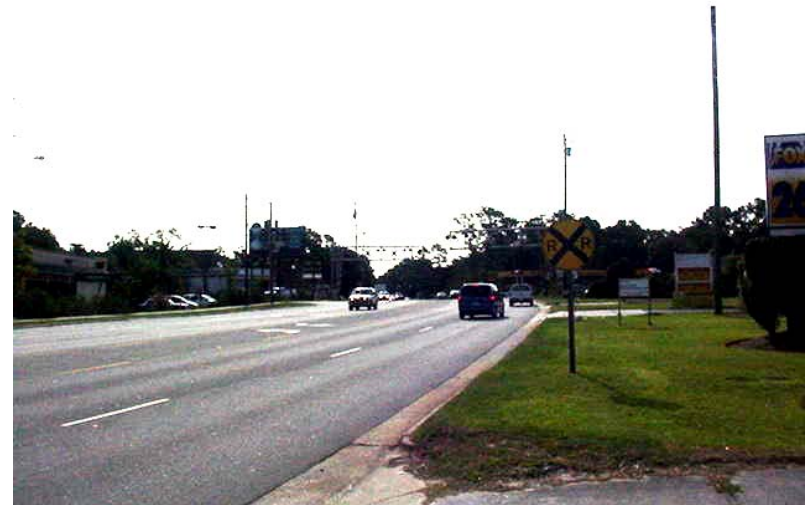
Image AA.1: View east from Dawson Street / Oleander Drive intersection. Lack of landscaping, street trees, and sidewalks.
