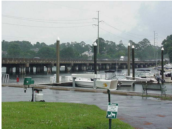
Image 9: Bradley Creek Bridge
