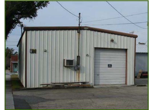
Building with full metal facade.
